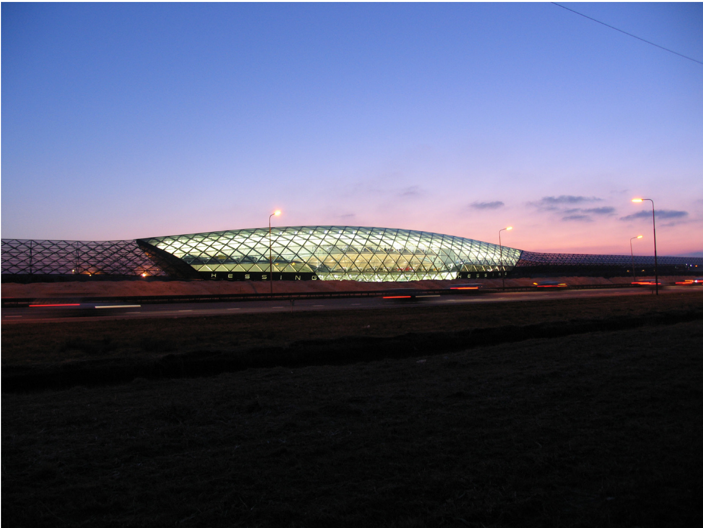
Figure 7. Cockpit in Sound Barrier (2005) A2 Highway Leidsche Rijn, Utrecht Architect ONL Source: ONL
